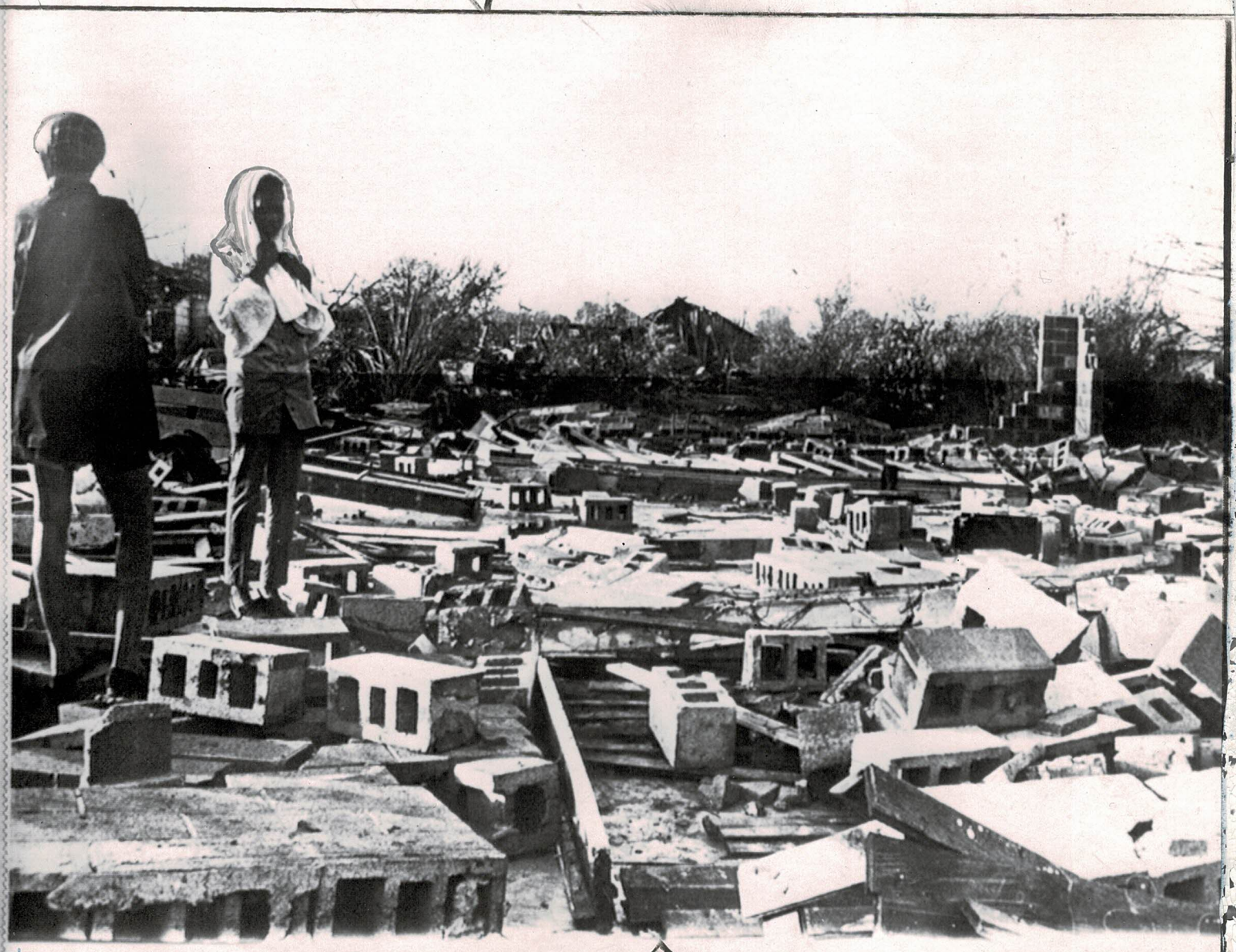
(MX2) CORINTH, Miss., April 20--WHERE TWO DIED--Scattered cement blocks were all that remained today of Triumph Sanctified Church in Corinth, Miss., following a tornado that smashed through the small city. Two of the five known dead and many among the dozens injured were inside the church when the twister struck on the heels of the Sunday morning service. (AP WIREPHOTO) (dss20054str) 1970
